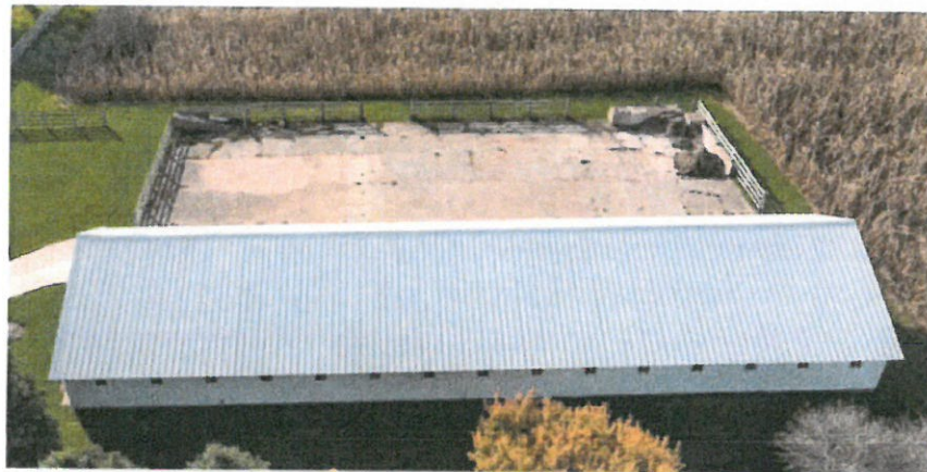
Back Elevation (North Facing)
